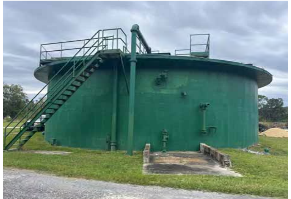
Sewer plant holding tank
