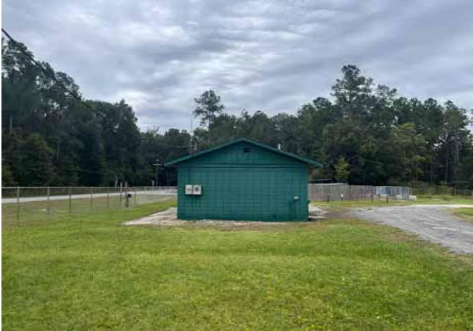
Sewer pump house
