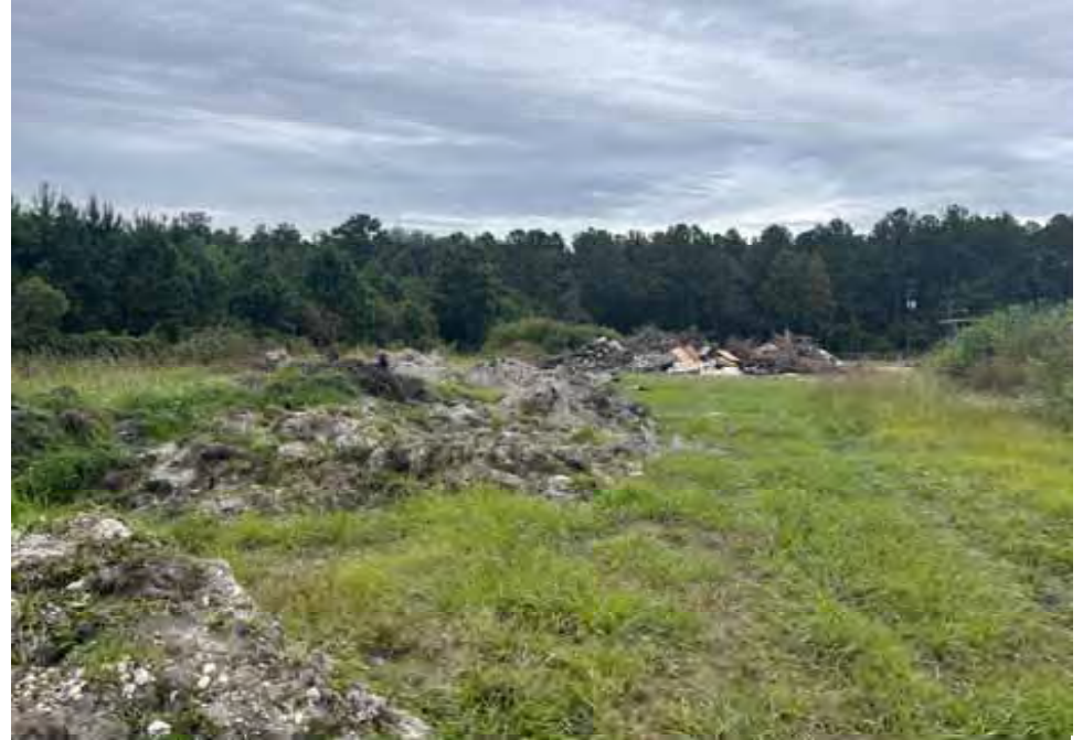
Dug pits with burnt wood and metal
