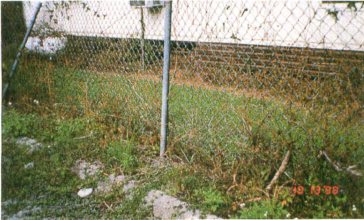
Photo E: Fenceline looking onto hospital property.
