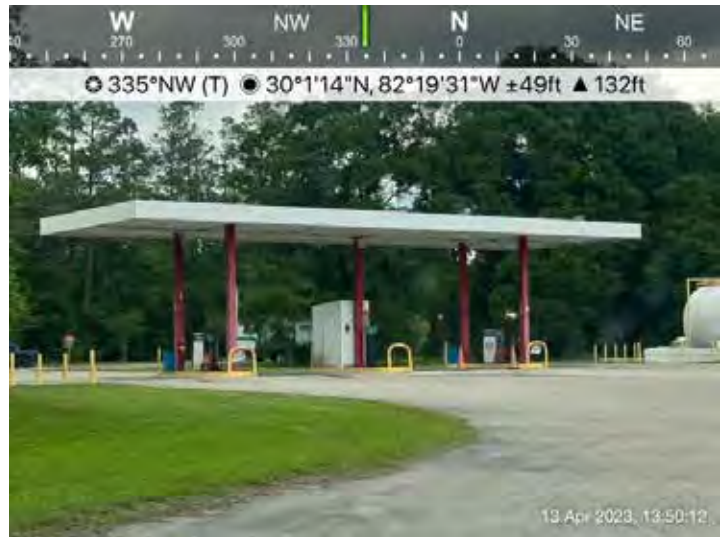
PHOTOGRAPH 8 Pritchett Trucking Fueling Station Pump Island and Canopy
