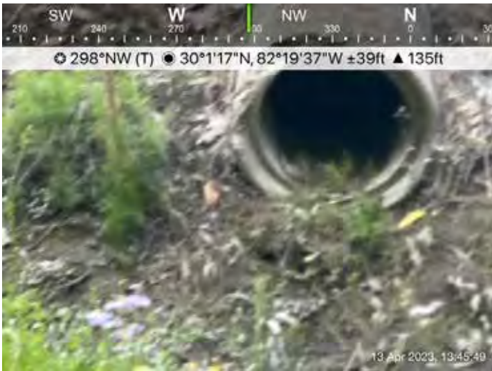
PHOTOGRAPH 3 Drainage Pipe on Subject Property
