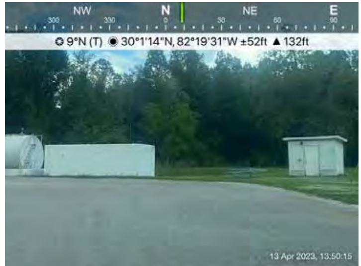
PHOTOGRAPH 10 Pritchett Trucking Fueling Station
