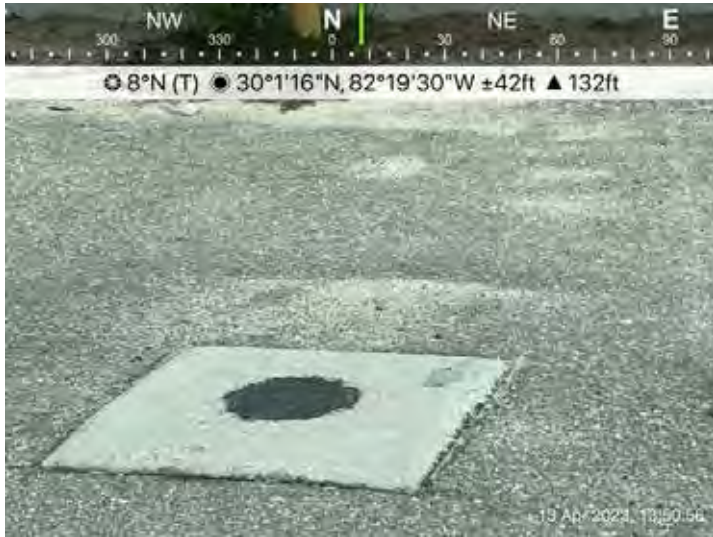
PHOTOGRAPH 13 Monitoring Well at Pritchett Trucking Fueling Station
